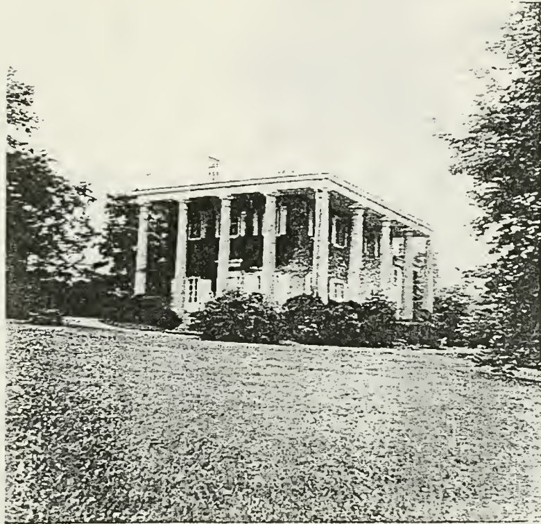
Figure 6: View of Wetherill addition, circa 1950
